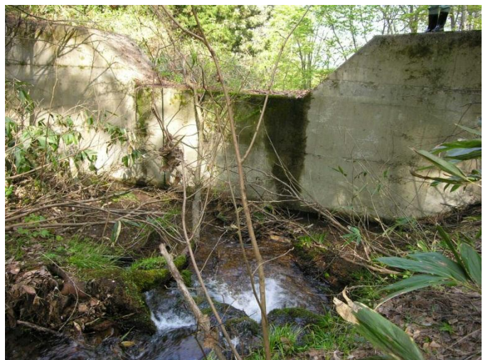
6 ③砂防えん堤
